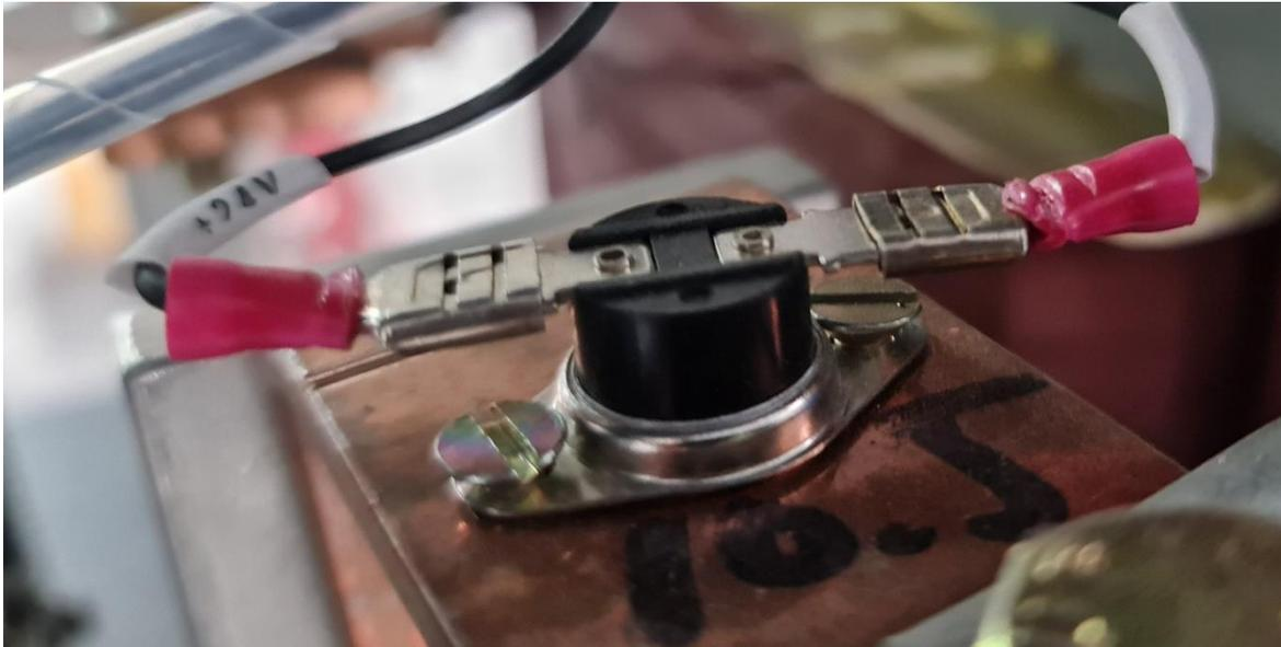
**Transformer Overload Protection & alarm**
